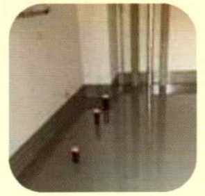
Epoxy Coating (Hospital inspection room)
