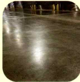
Concrete surface reinforcement (Logistics warehouse)
