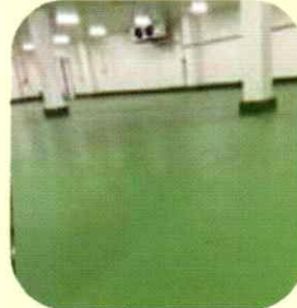
Water-Base hard urethane Coat (Logistics warehouse)
