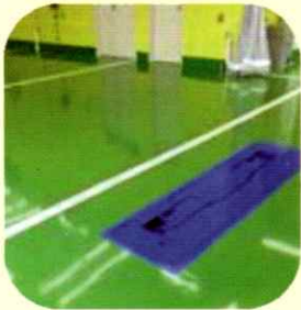
Epoxy coating (Car maintenance Shop)
